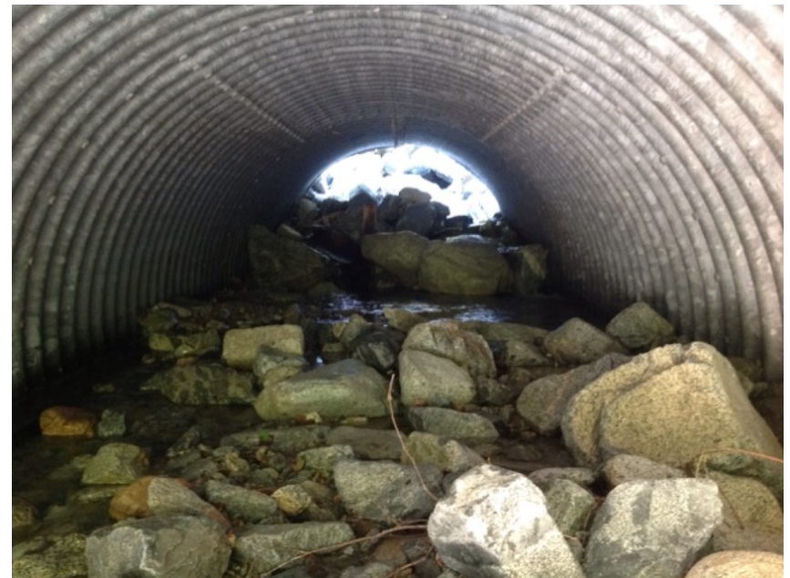
looking through culvert
