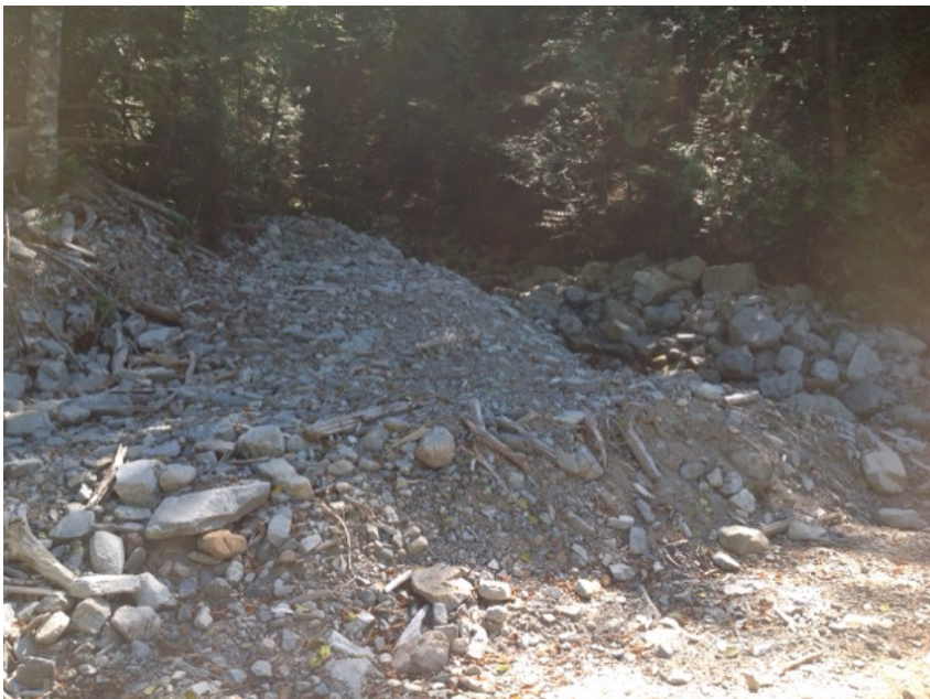
evidence of recent heavy flows
